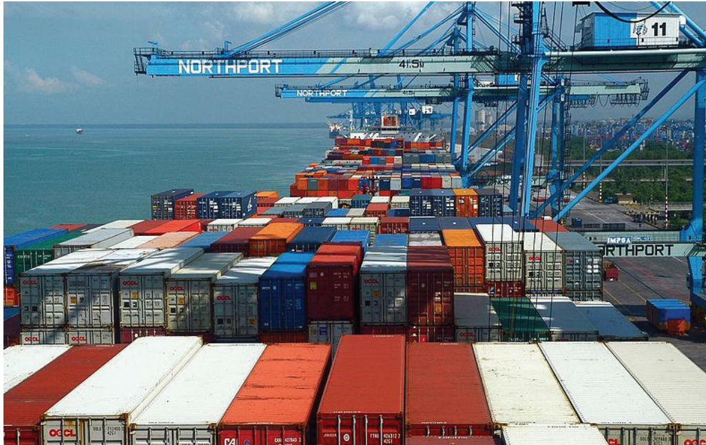
Containers at Northport (Port Klang), Malaysia
