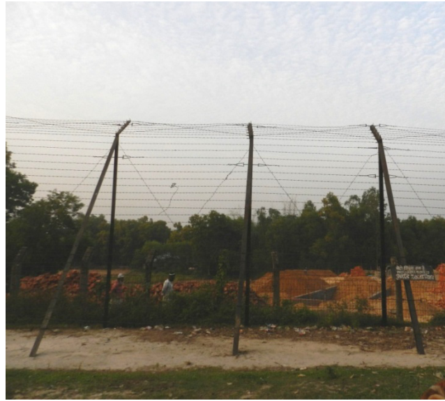
Kamasagar Border haat construction underway.
