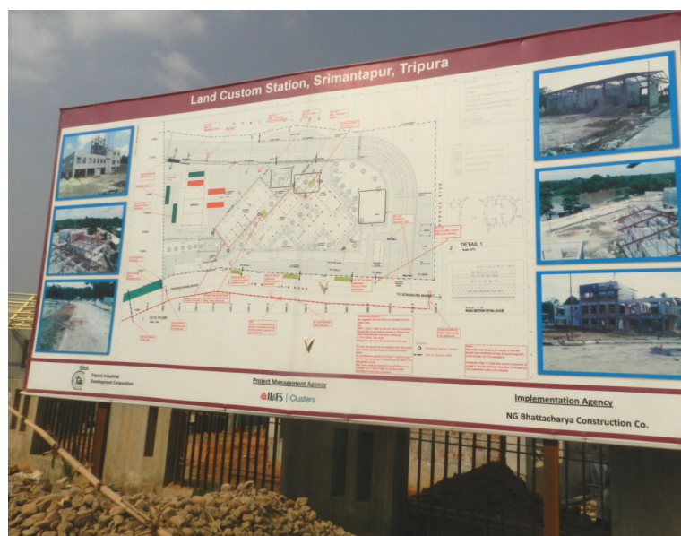
Construction underway at Land Customs Station, Srimantapur, Tripura, India.
